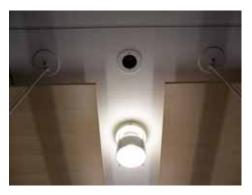
Several video sources are available in both the local presentation and videoconferencing modes. An Extron MGP-464 Quad Video Processor was installed allowing the end user to display up to four images on the screen simultaneously. Two ClearOne ceiling document cameras were provided enabling the ability to share clear color objects from multiple locations around the table.
